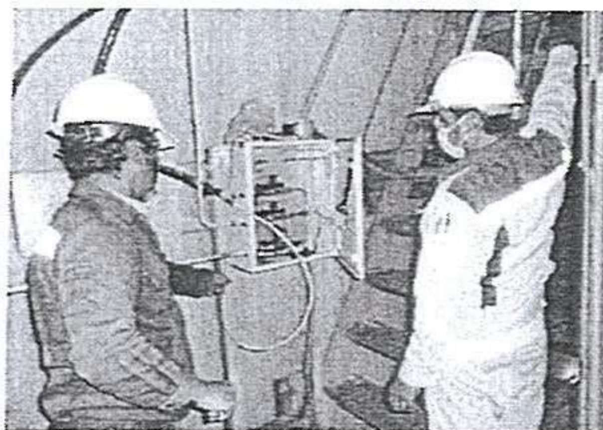
Flushing Sampling tube for Heated line stack1,2
