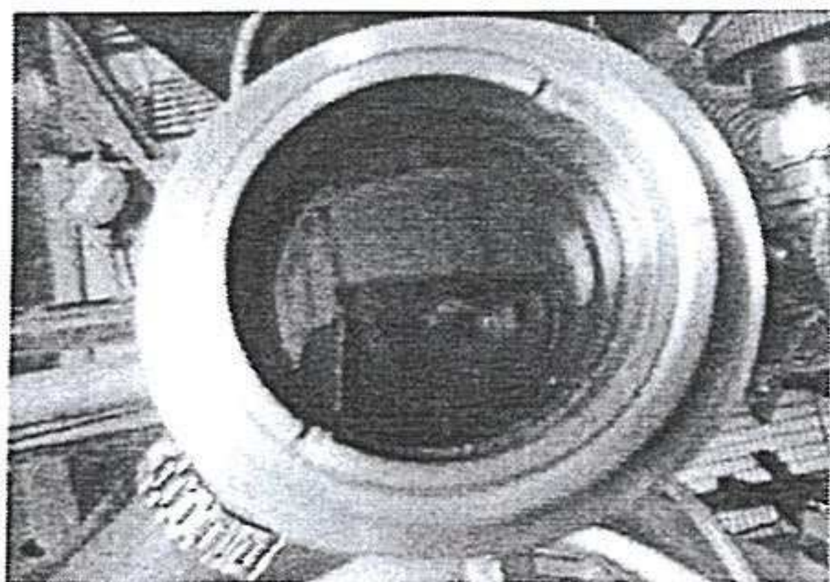
Cleaned lens for HCL sensor probe stack 2
